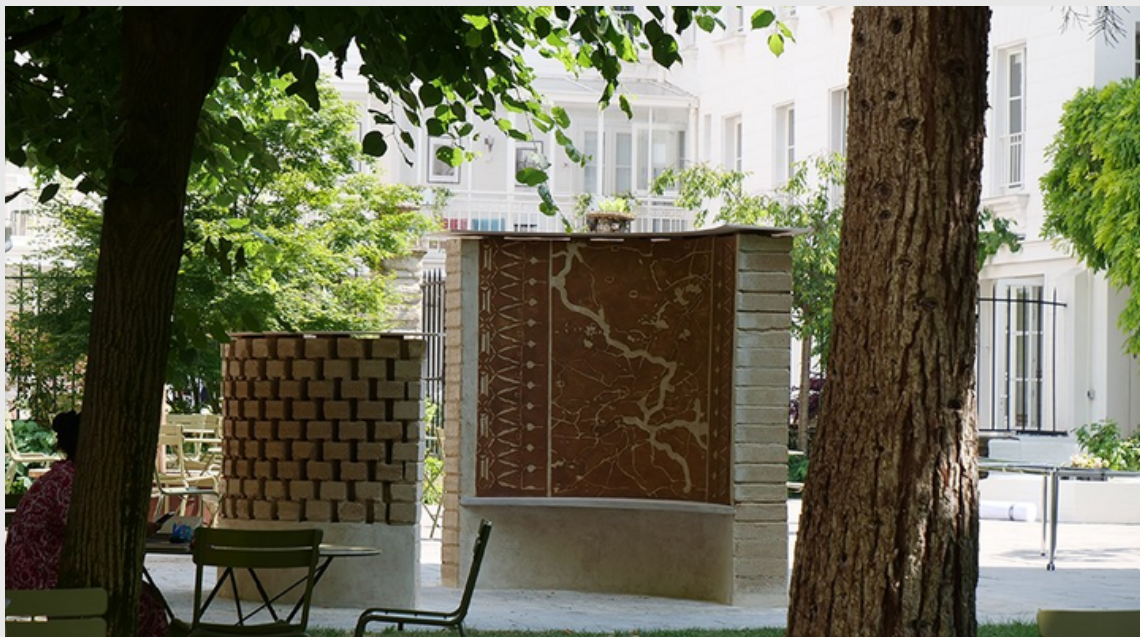
The Raw Earth Sgraffito Pavilion inaugurated at Reid Hall in May 2023 made entirely from materials sourced in Paris
